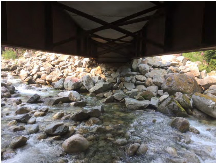
Left Bank Abutment when facing downstream
