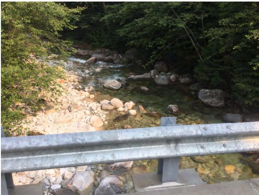
Looking downstream from deck
