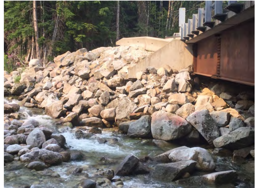
Steep riprap at left upstream
