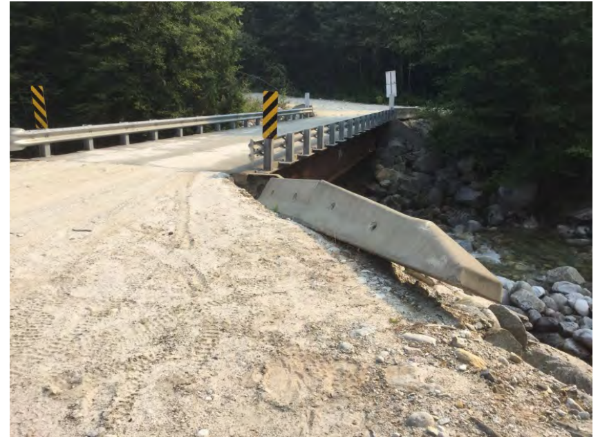
Failing left upstream no post barriers
