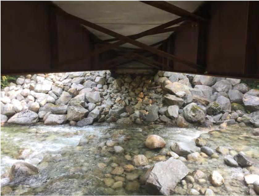
Right Bank Abutment when facing downstream
